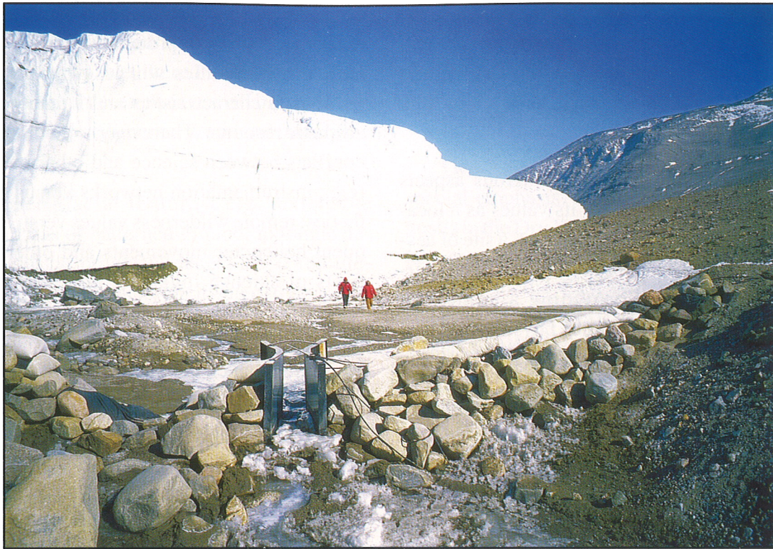
Weirs have been placed on many of the streams of the Dry Valleys by NZAP and USAP scientists to gauge the flows as a monitor of climate change and to estimate the flux of materials into the lakes.
